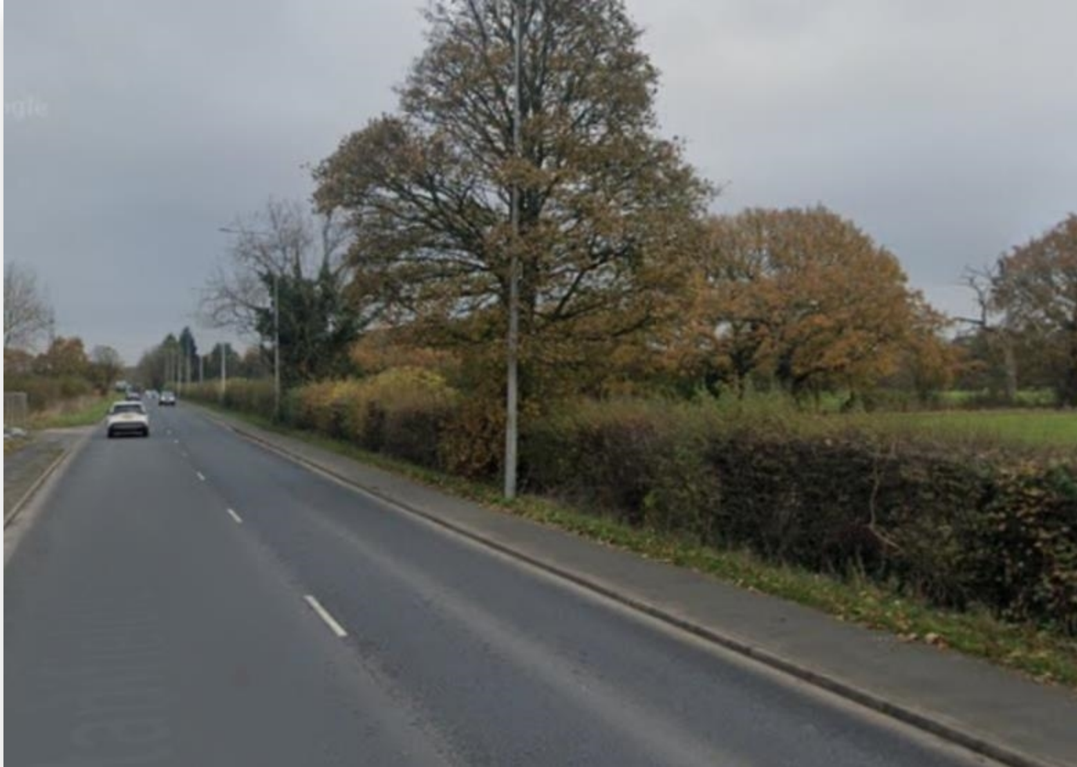
Stanifield Lane at Zone D
