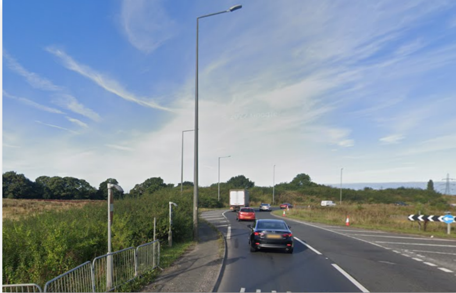
Approach to the M65 terminus roundabout
